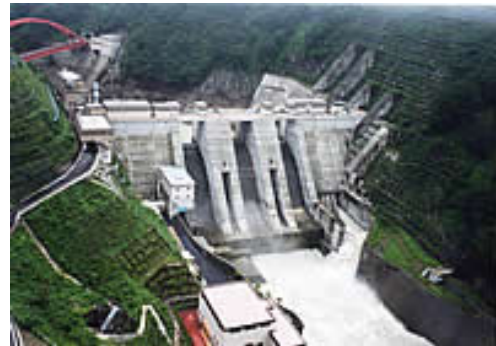
Figure 3 Combination flushing of the Unazuki Dam in the Kurobe River(June, 2001)
